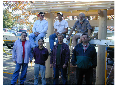
Japanese Gate and Volunteer Timber Framers
